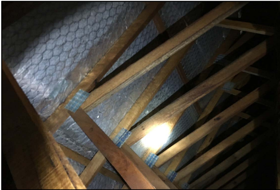
Photo 7: Building 3 - Sarking (entire roof area) insulation lining under roof
