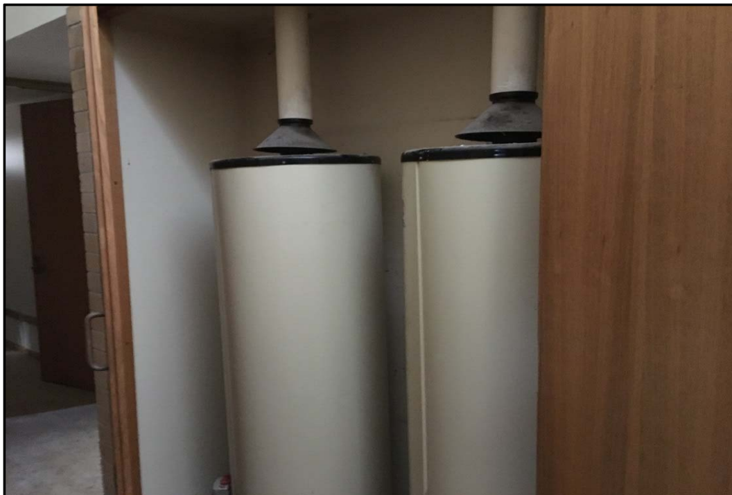
Photo 2: Building 3 - Cement Flue Pipes – Hot Water System
