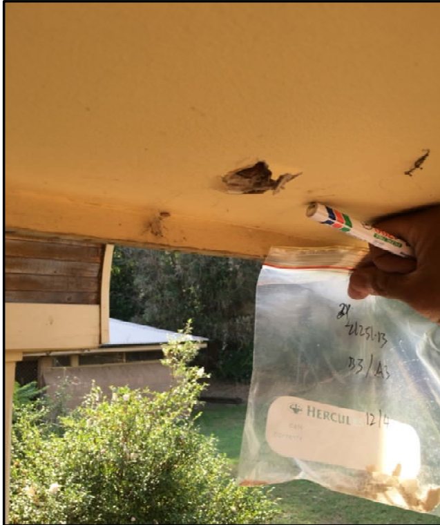
Photo 1: Building 3 - Fibrous Cement Sheet Eaves
