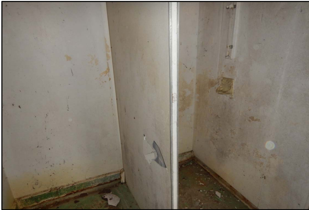
Photo 12: Building 7 - Vertical cement sheeting dividers in shower
