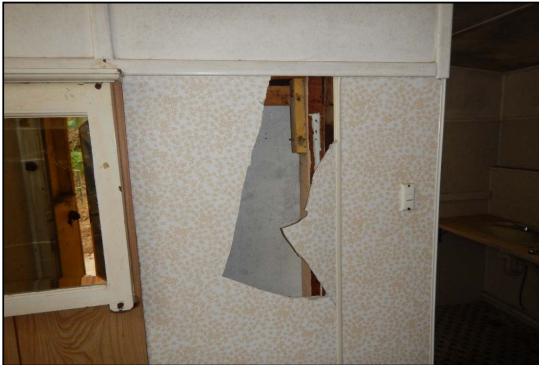
Photo 10: Building 7 - Patterned cement sheeting in bathroom
