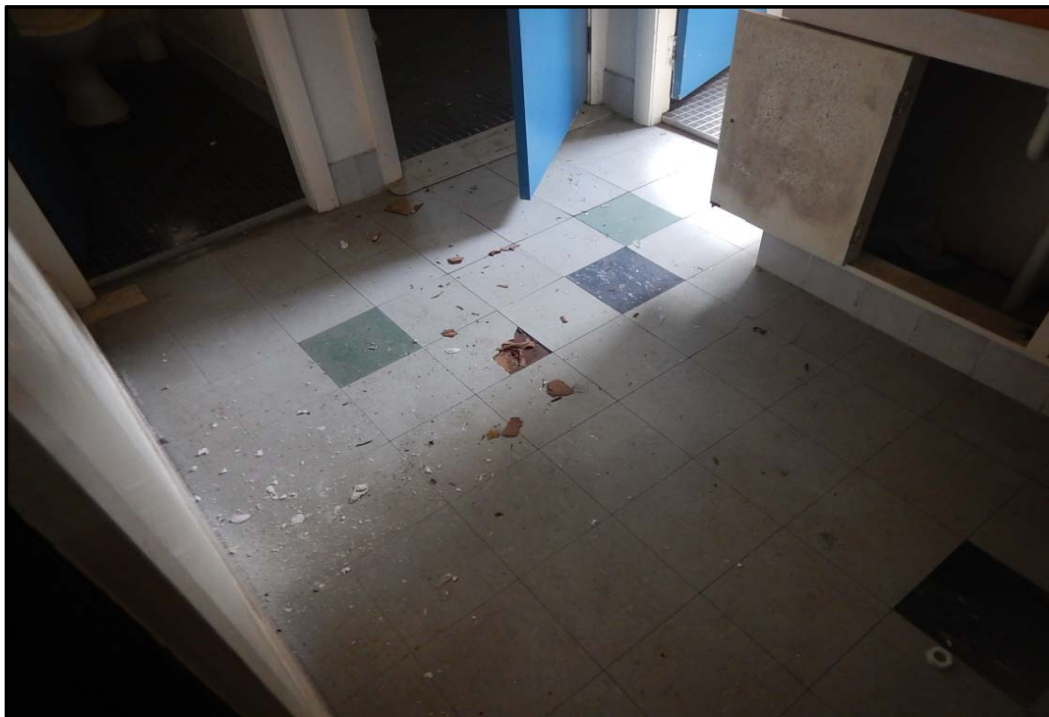
Photo 16: Building 8 - Grey vinyl floor tiles in bathroom
