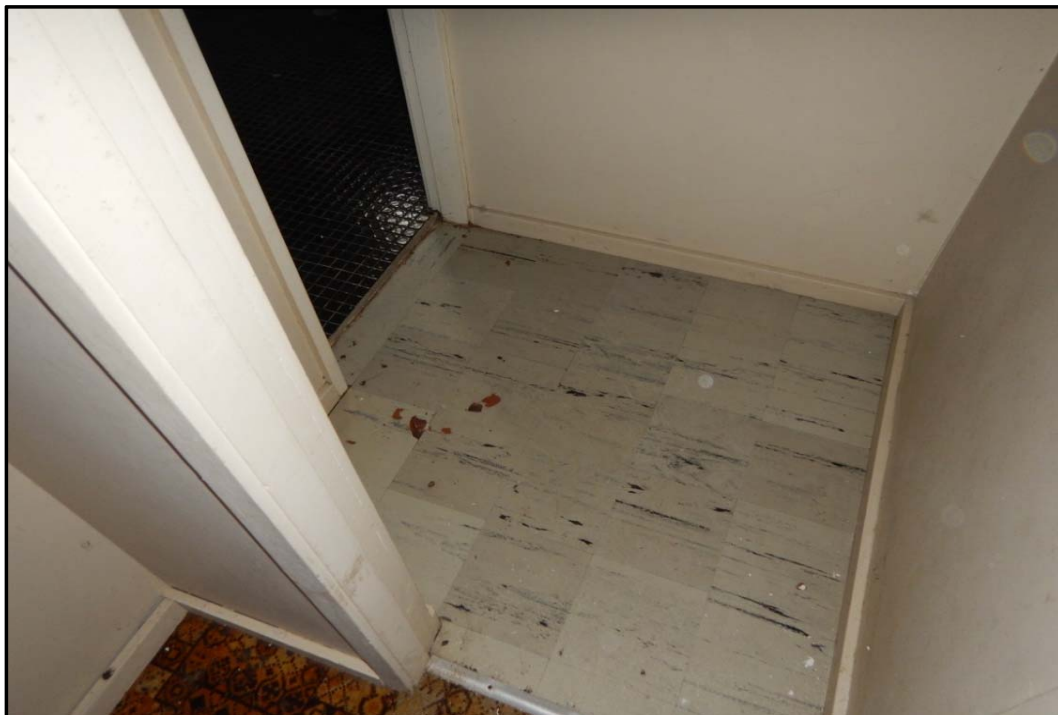
Photo 18: Building 8 - Light grey vinyl tiles in main bathroom
