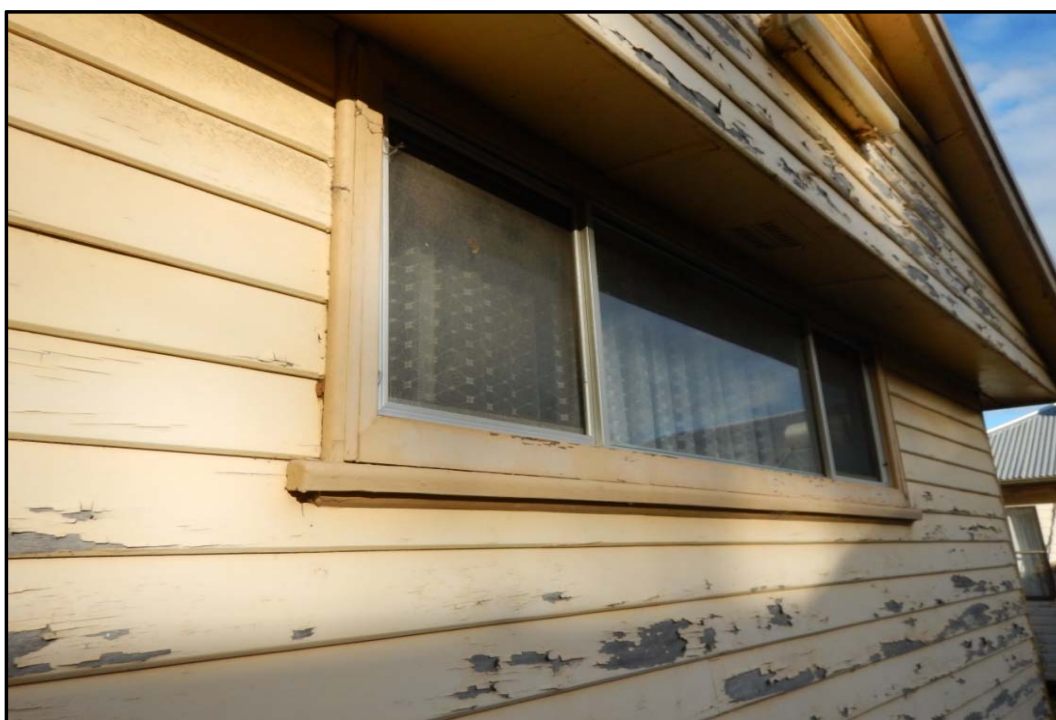
Photo 25: Building 9 - Dark yellow paint on window frames and sills
