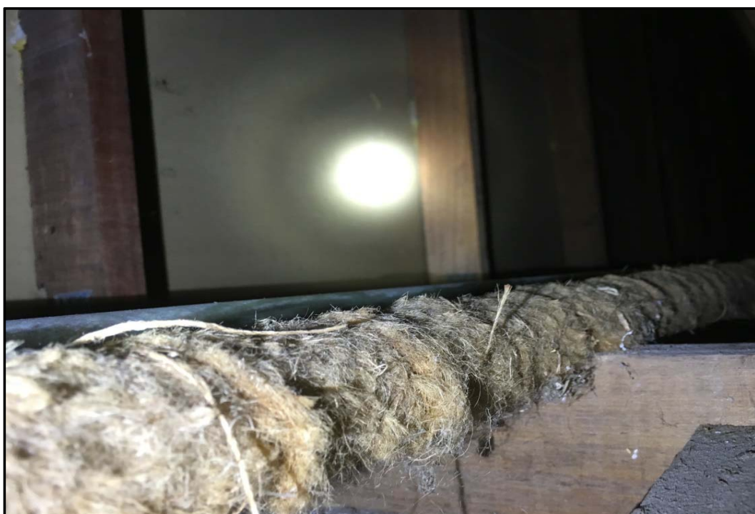
Photo 6: Building 3 - Roof void – Brown fibre lagging around pipe
